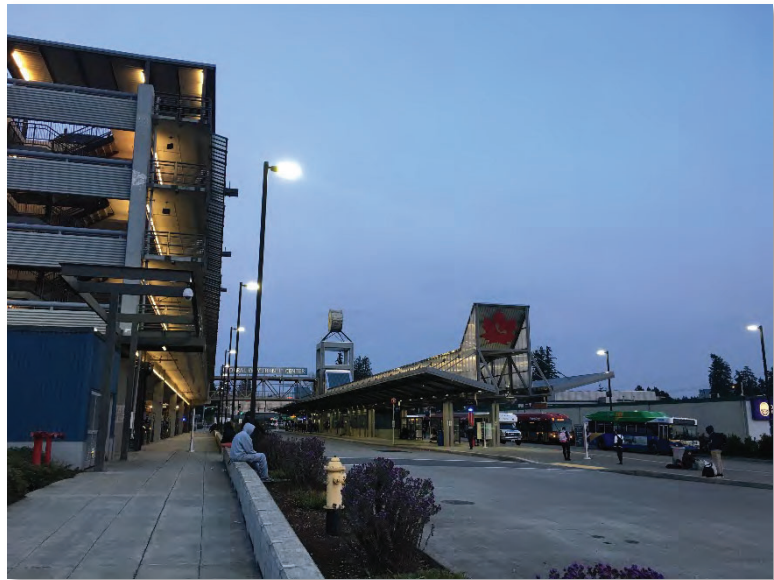
The Federal Way Transit Center in downtown Federal Way (Courtesy of the Volpe Center)
