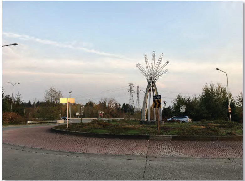
This roundabout services an on-ramp to I-5 on the northern end of downtown Federal Way (Courtesy of the Volpe Center)
