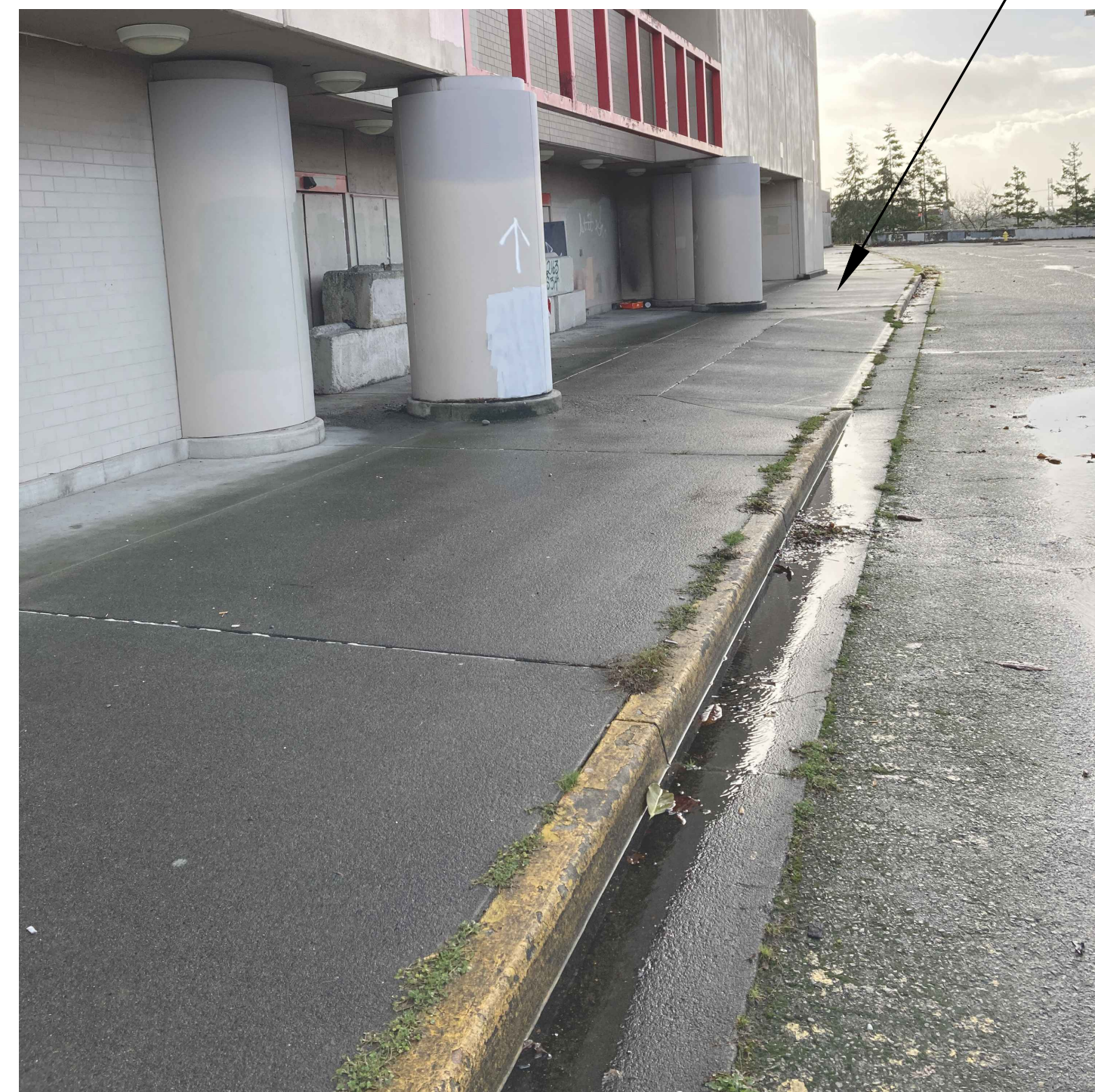
WEST SIDE WALKWAY REMOVAL
