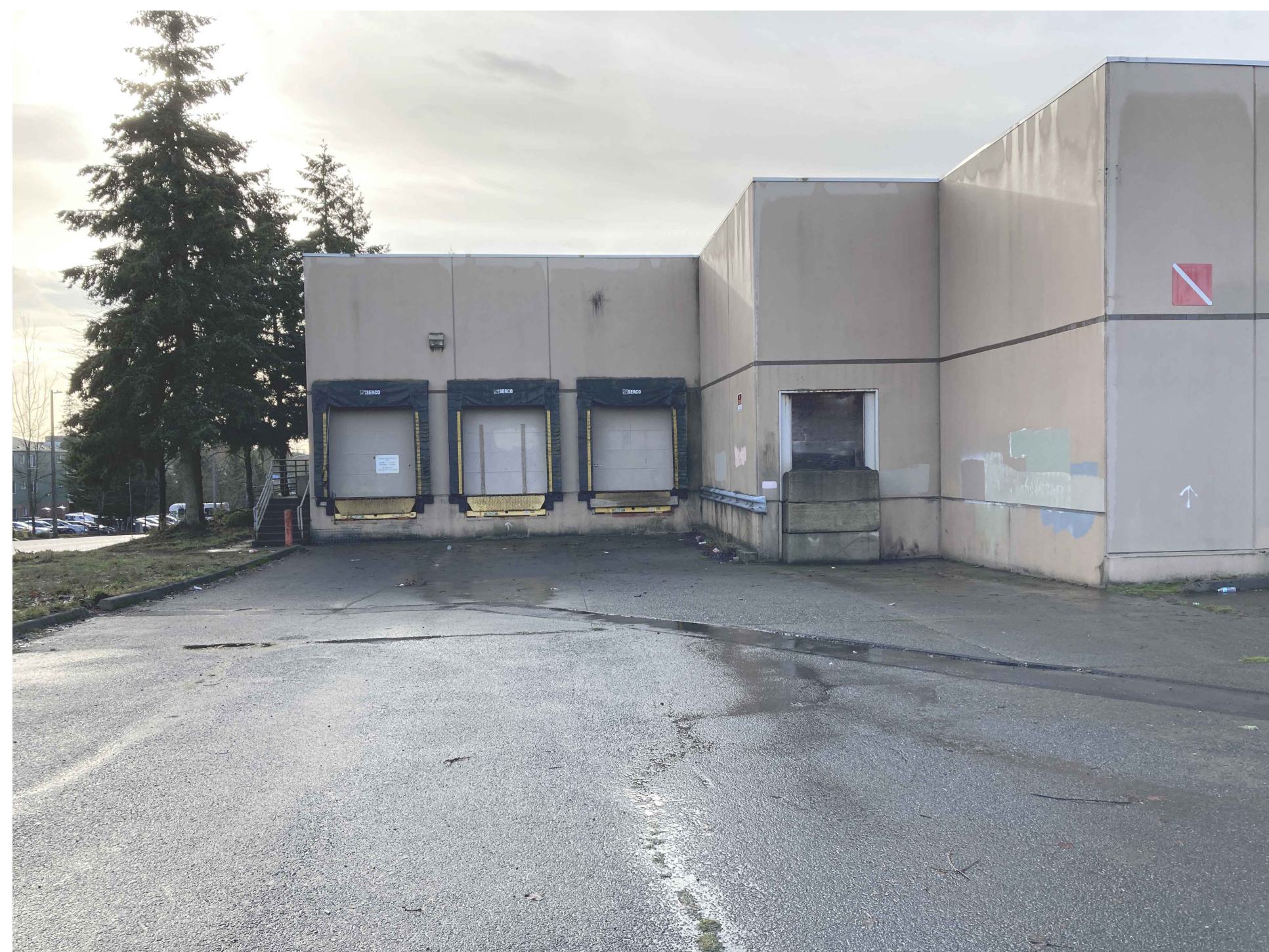
NORTHEAST LOADING DOCK
