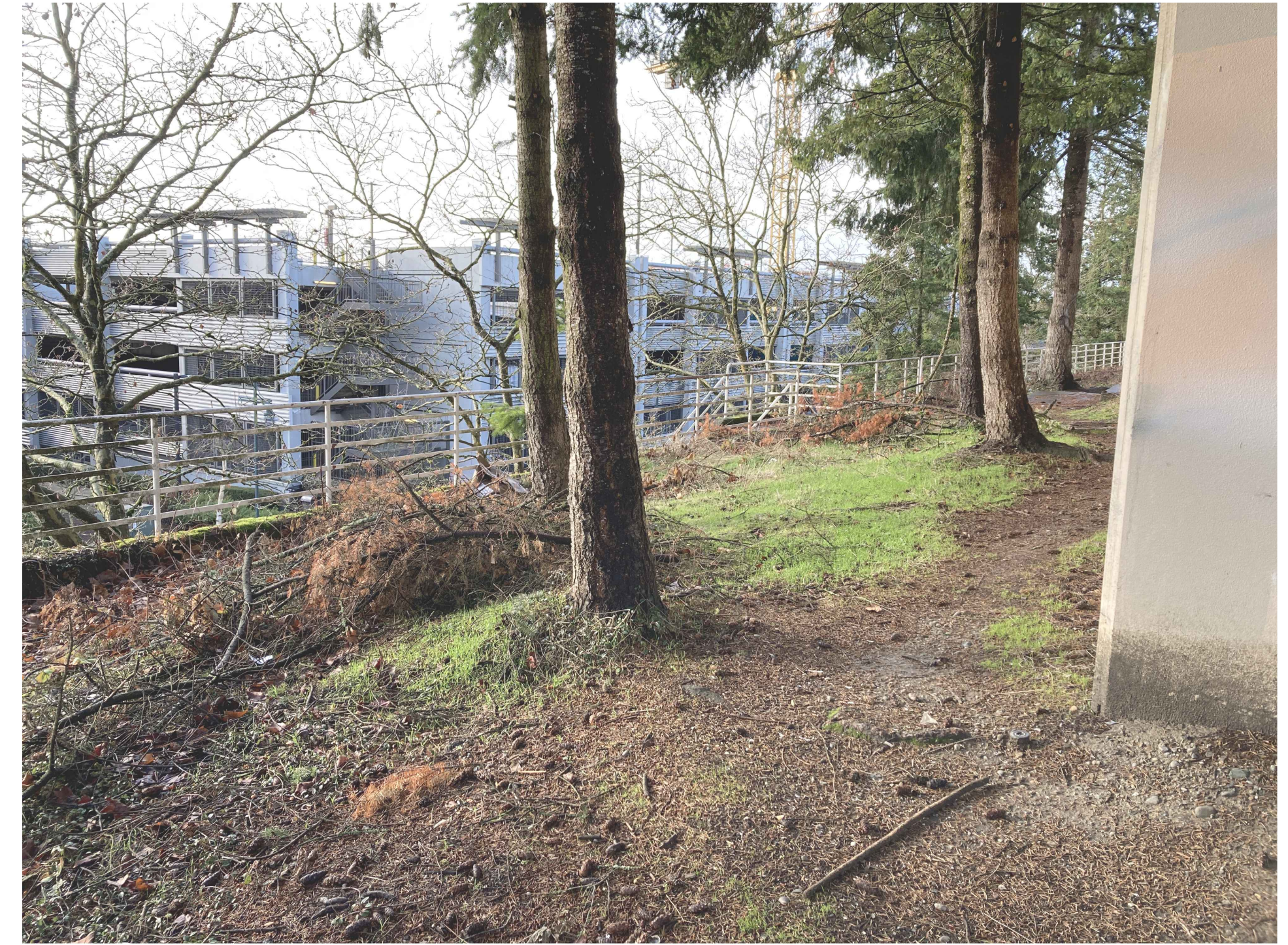
SOUTHEAST CORNER, WALL & RAILING
