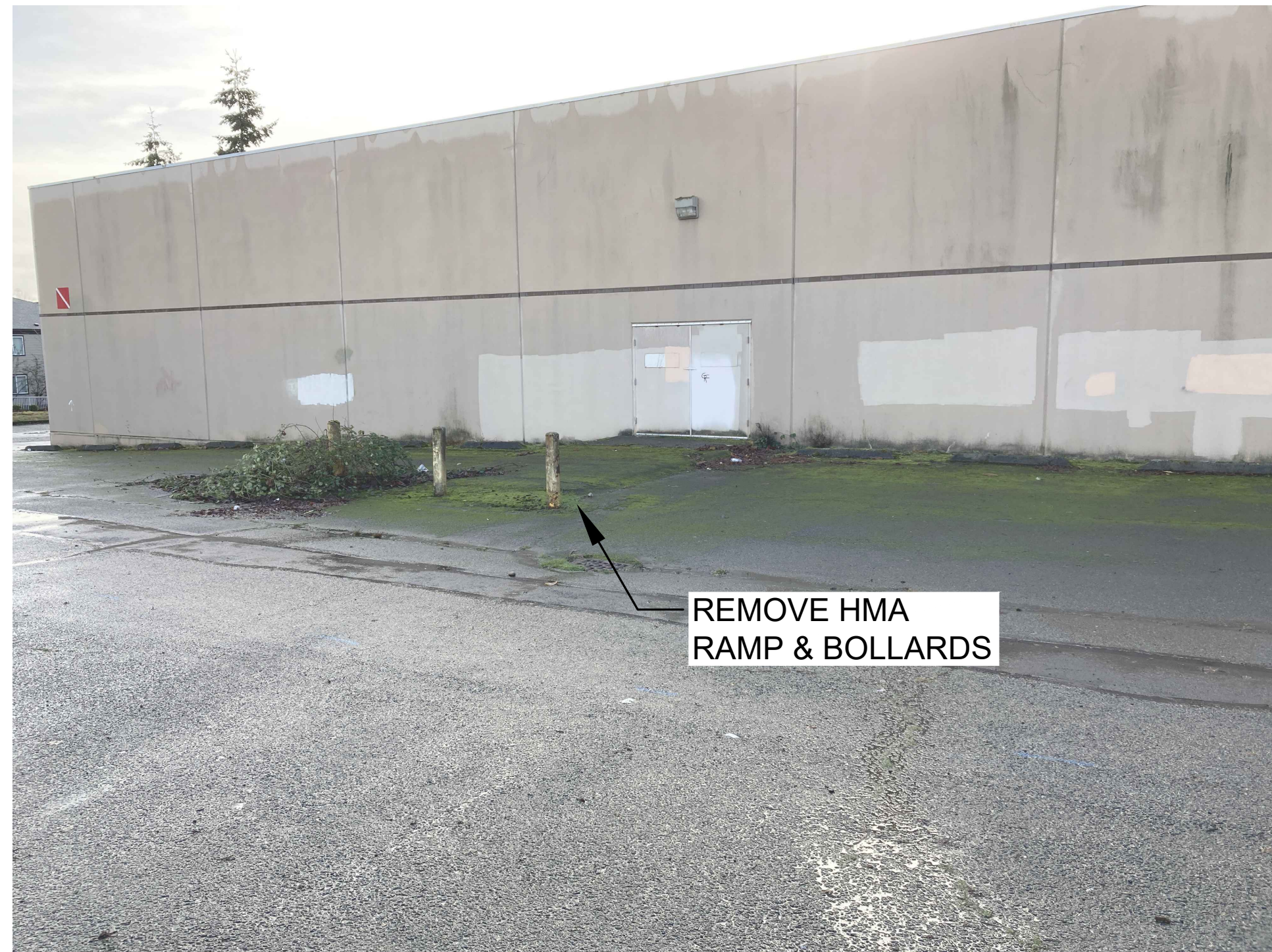
NORTH HMA RAMP REMOVAL
