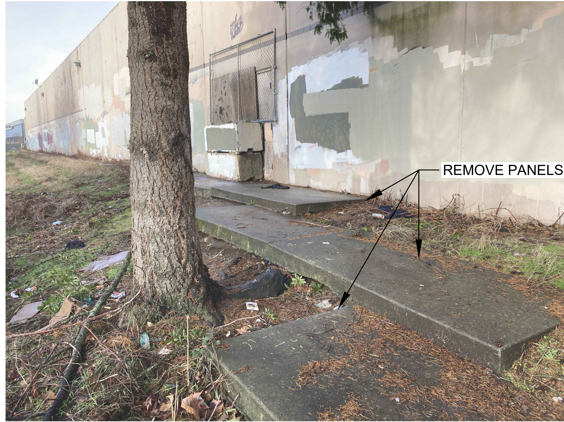
SOUTHEAST WALKWAY REMOVAL
