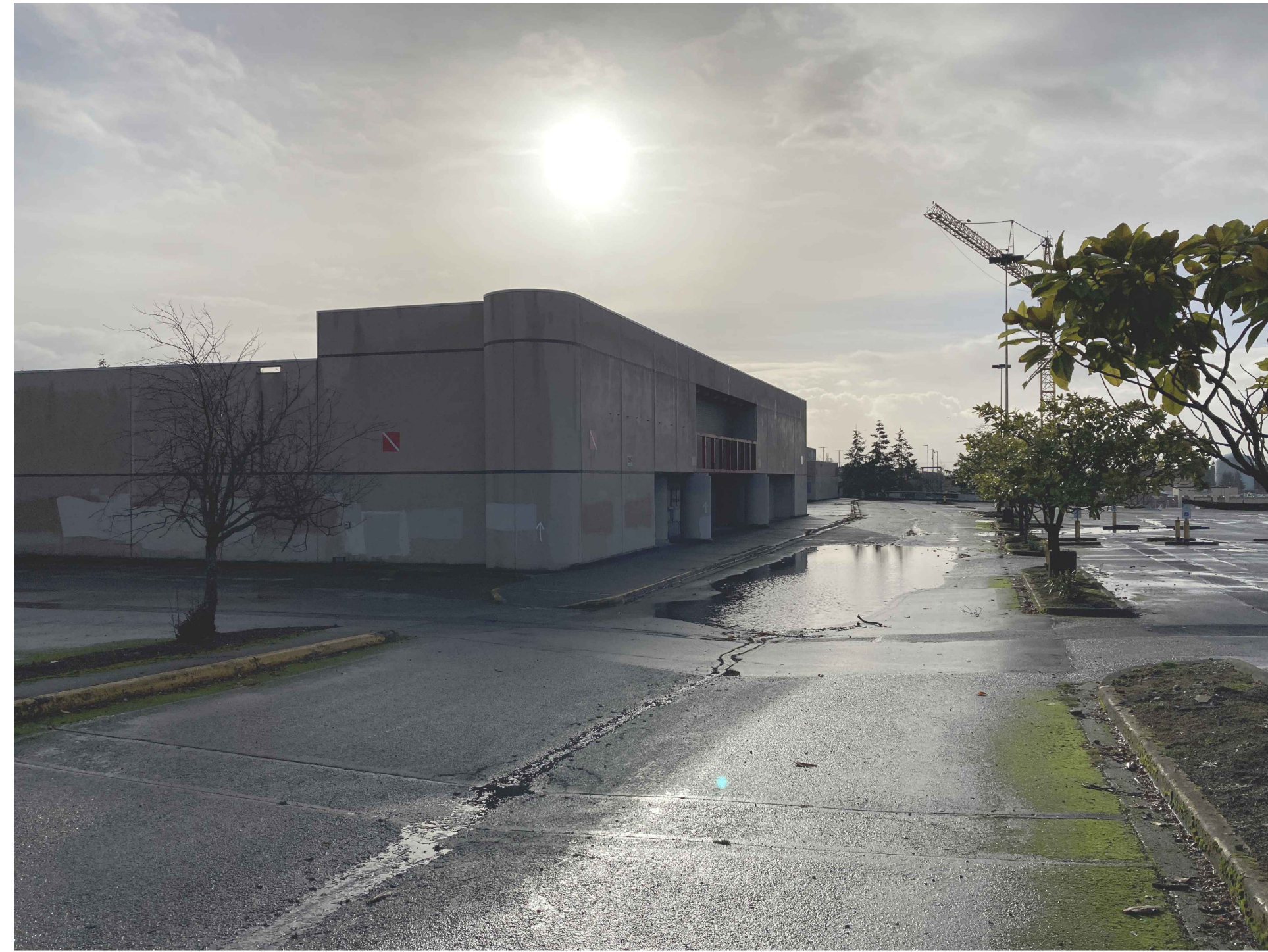
MAIN DRIVE AISLE
