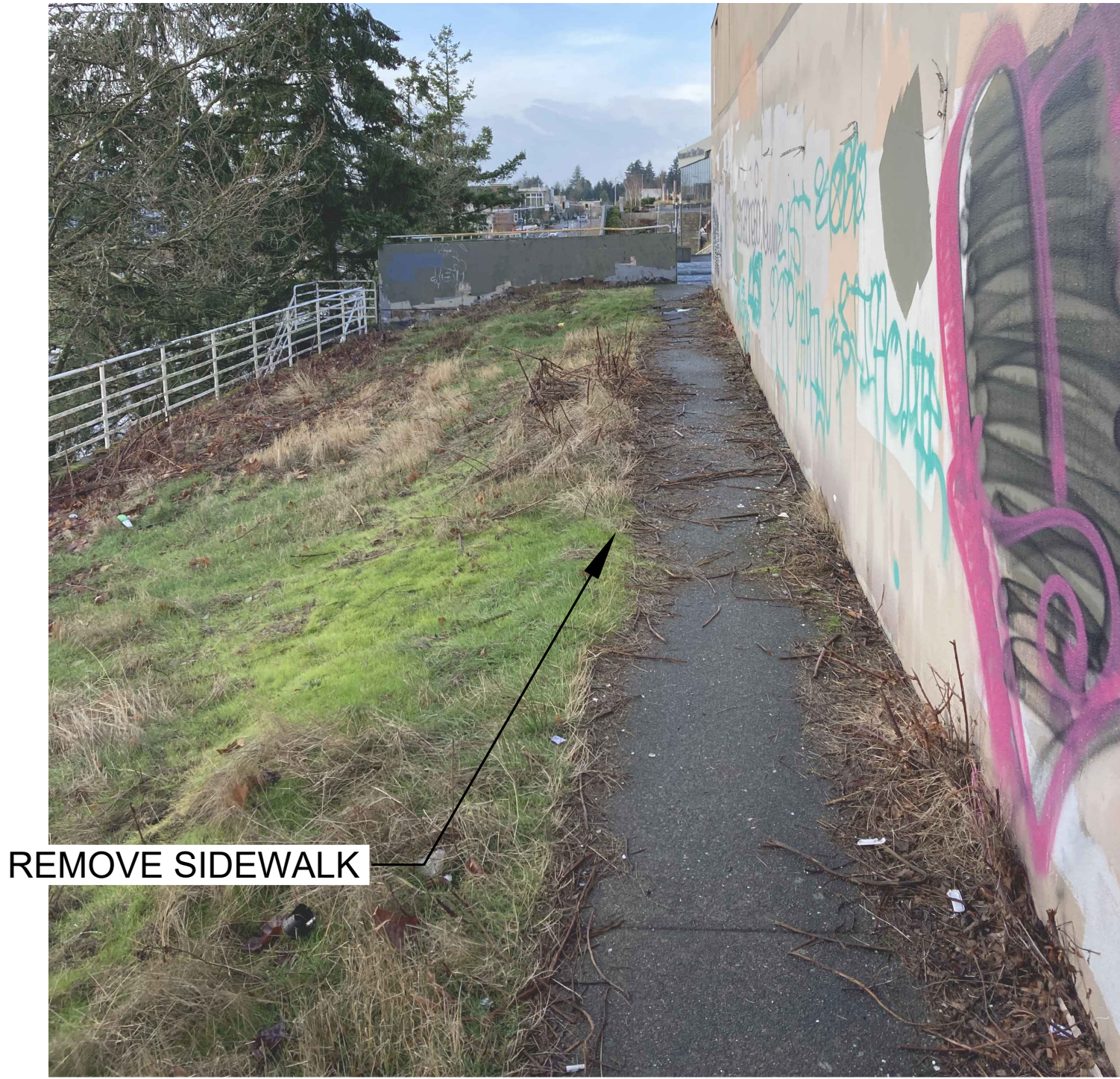
SOUTH SIDE BUILDING (FACING WEST)
