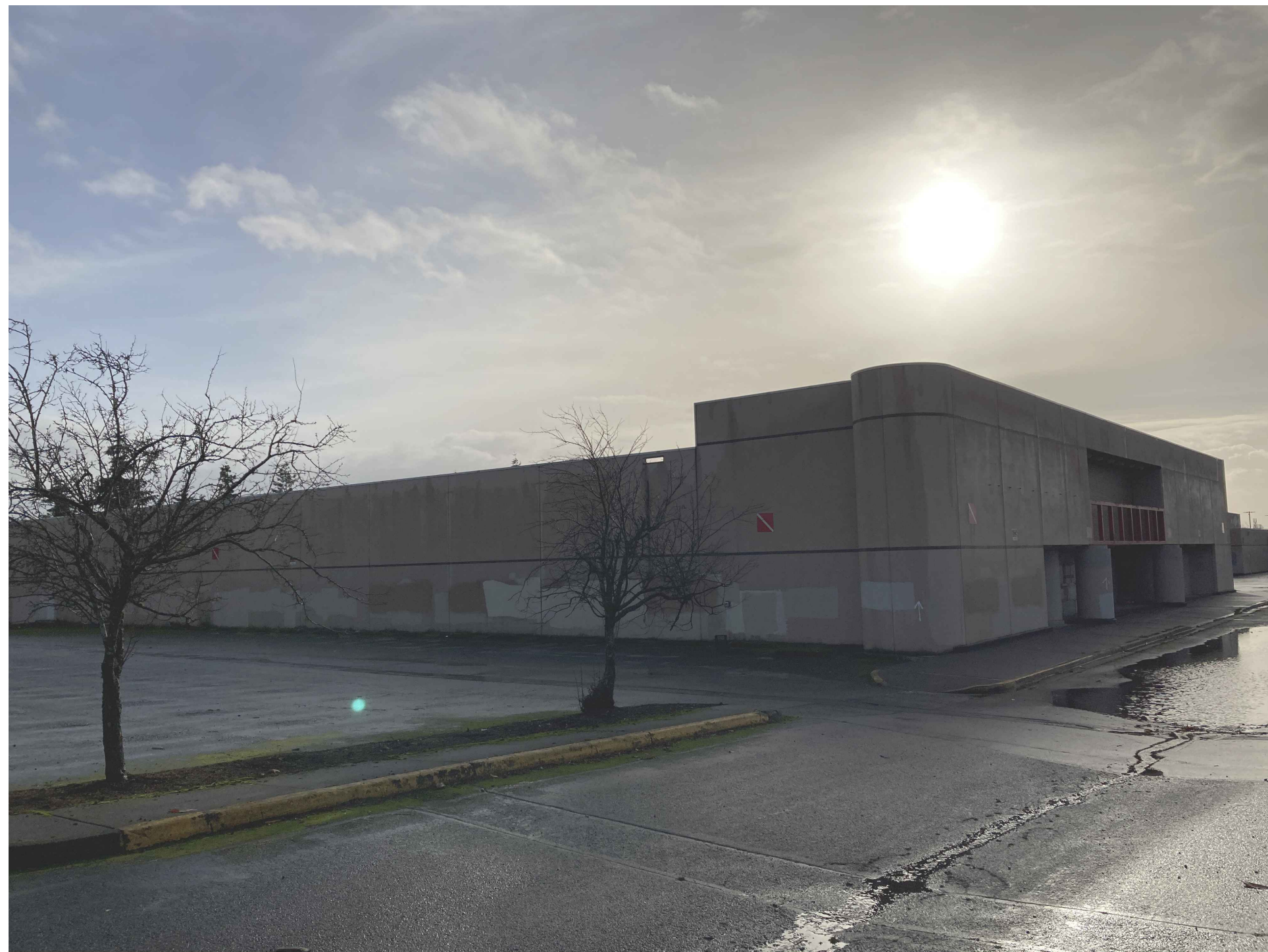
NORTHWEST BUILDING CORNER
