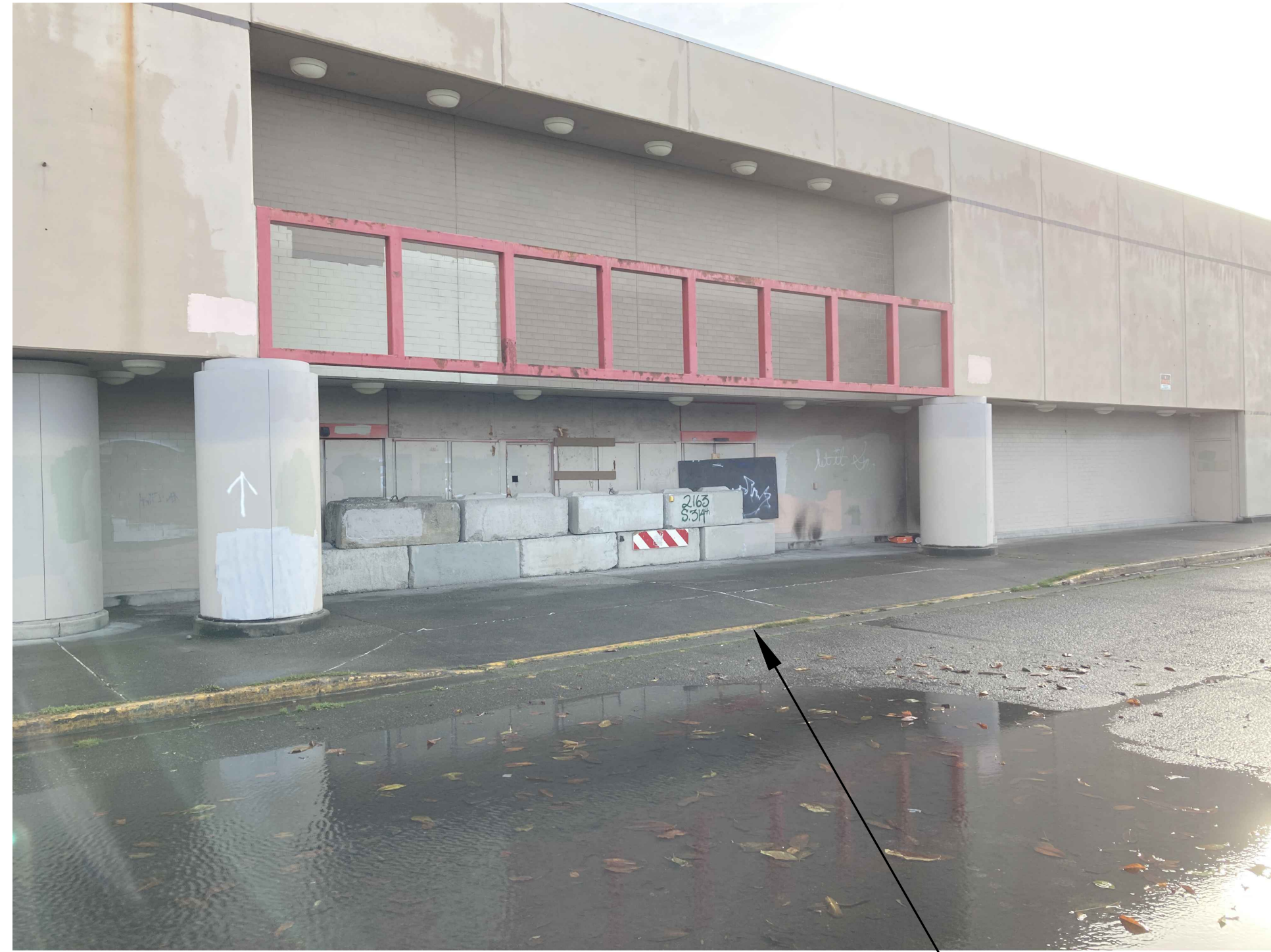
WEST SIDE BUILDING
