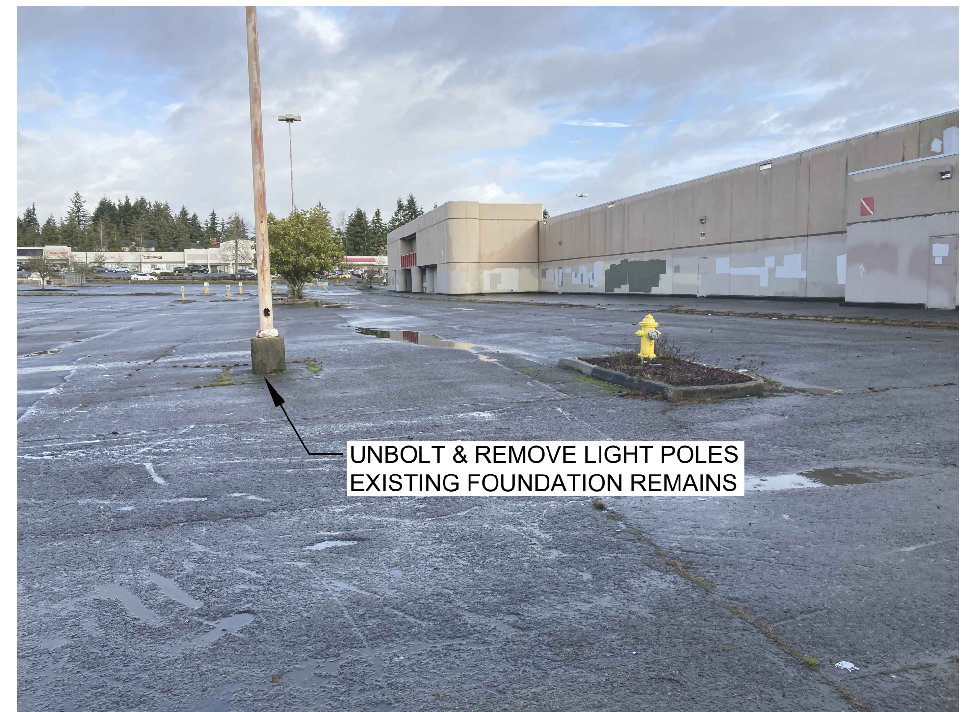
SOUTHWEST PARKING LOT (FACING NORTH)
