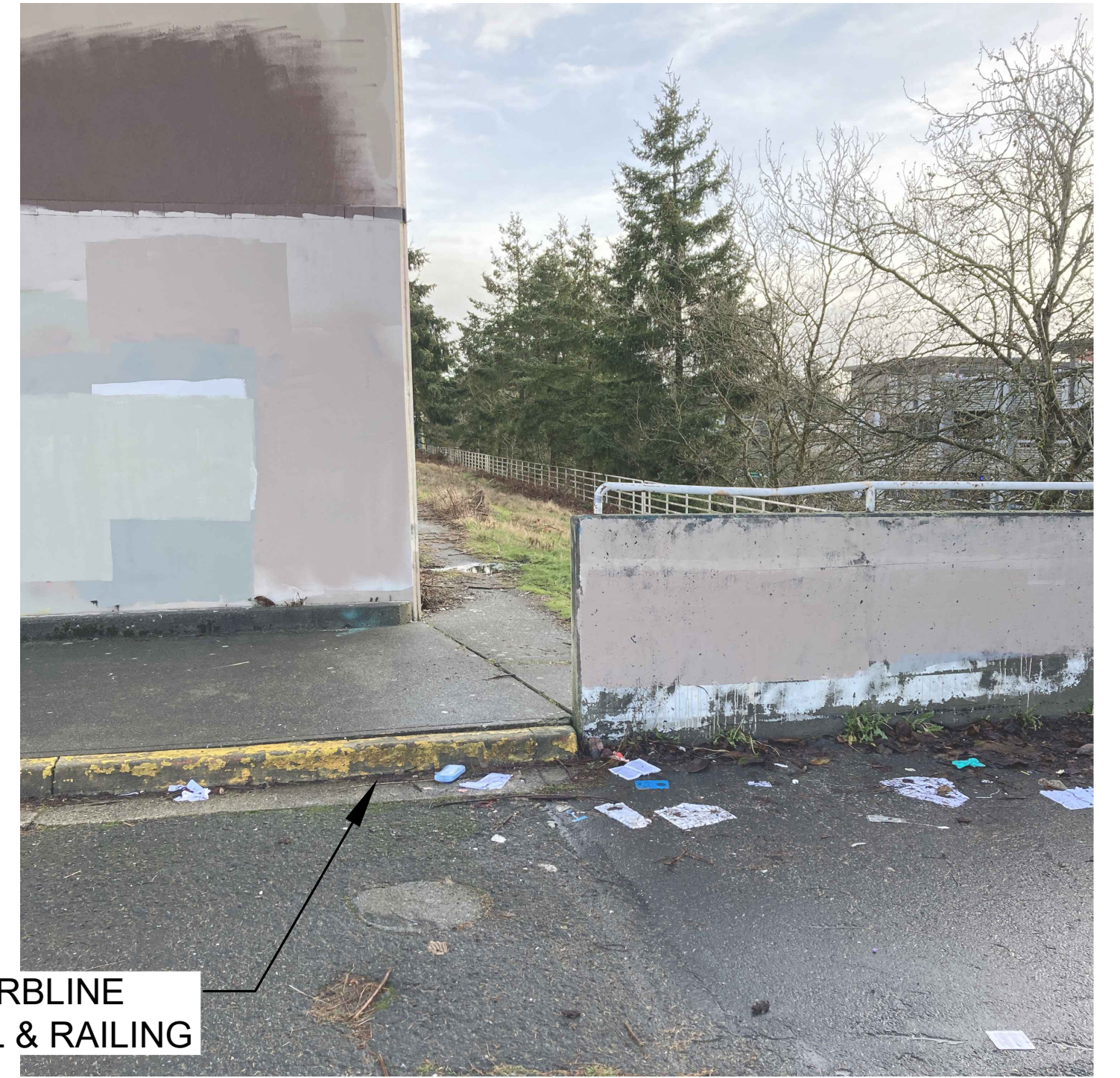
SOUTHWEST CORNER, WALL & RAILING
