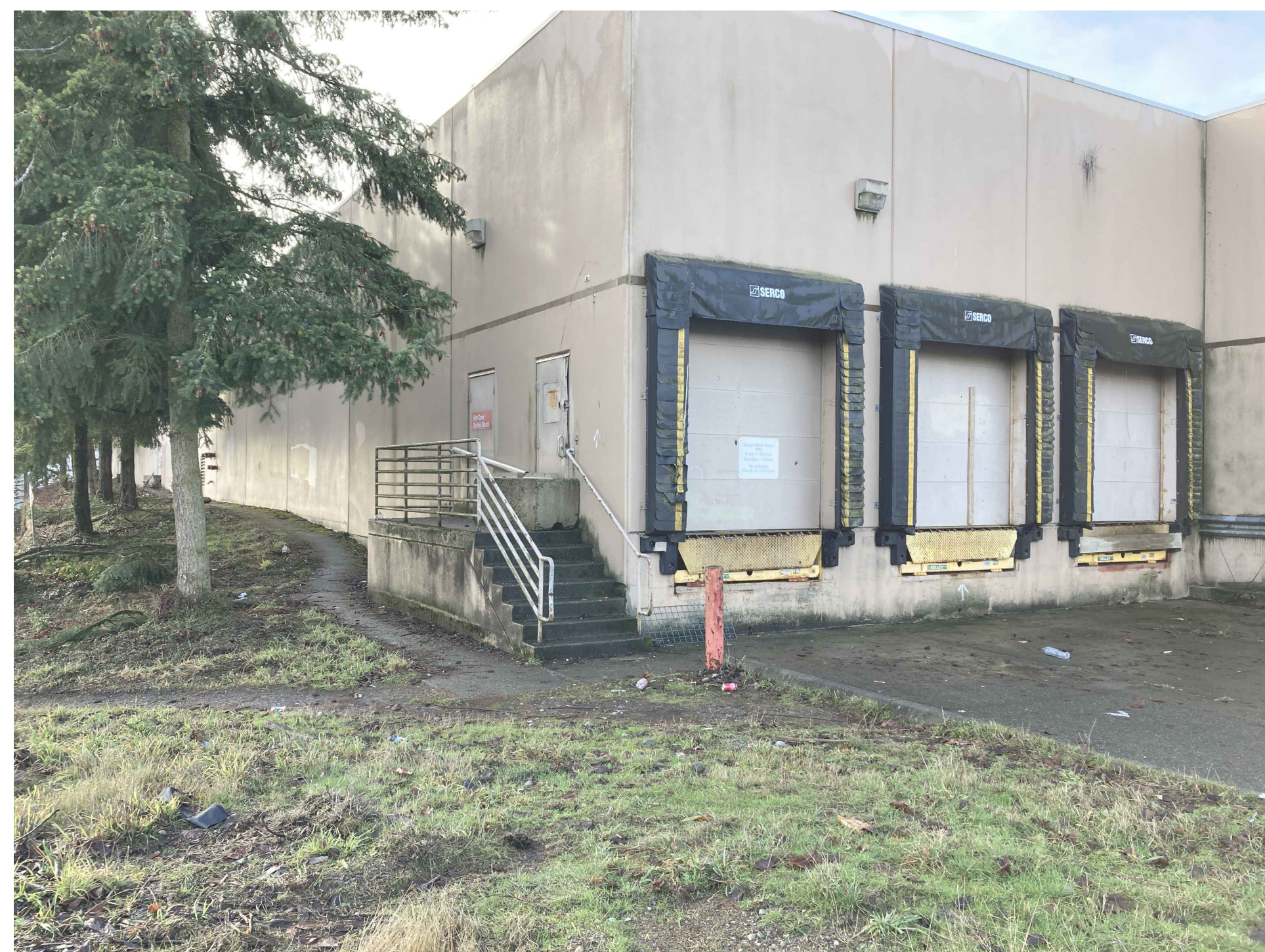
NORTHEAST BUILDING CORNER
