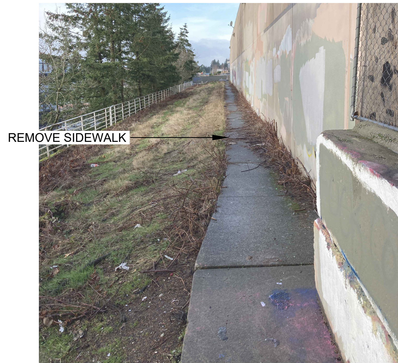
SOUTH SIDE WALKWAY REMOVAL
